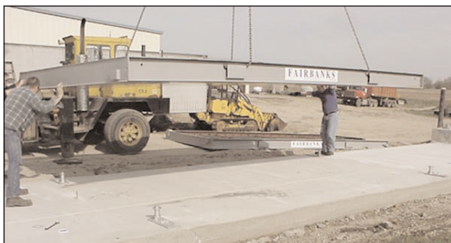
Fairbanks' RC Field Pour Series truck scales feature light-weight, easy-to-install modules.
